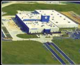
PAGELAND, SC Bronze Foundry and Manufacturing Plant
